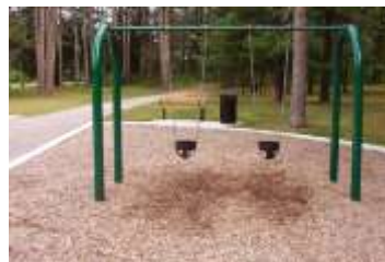
Engineered wood mulch base with concrete curb
